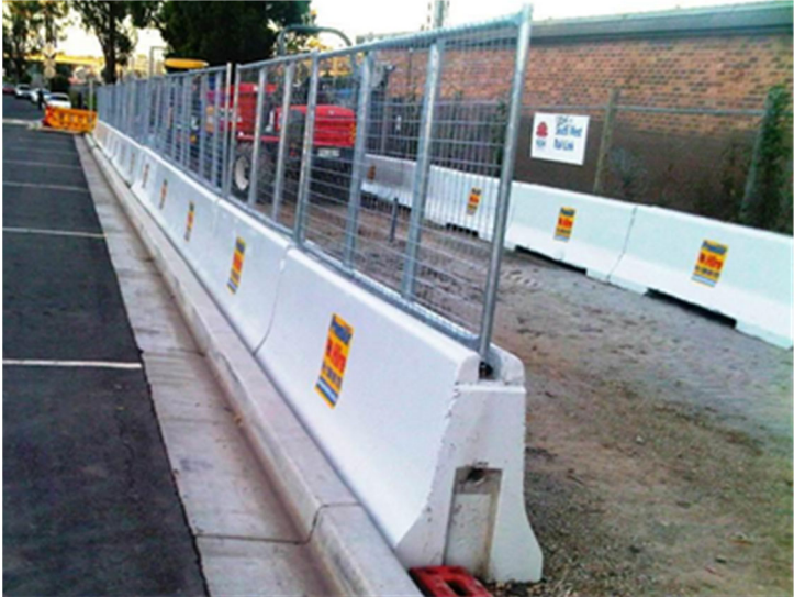
Image 2 – kerbside concrete barrier
