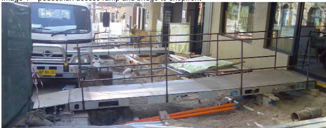
Image 1 – pedestrian access ramp and bridge to shopfront
