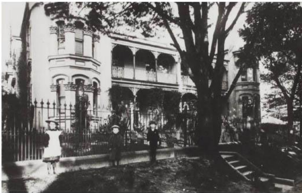
Figure 5: Banksia and Wytchazel behind an original iron palisade fence, reinforcing the "private street" nature of this entry to the site. (Source: Vickery Album, SLNSW, PXA 1742)
