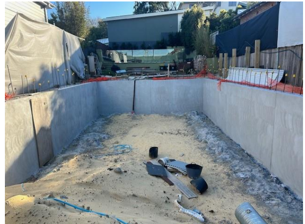
Figure 2: Excavated basement level with capping beams at side, facing north
