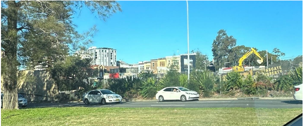
Figure 3: Site as viewed from Syd Einfeld Drive, looking south-east
