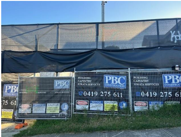
Figure 1: Site frontage, facing north
