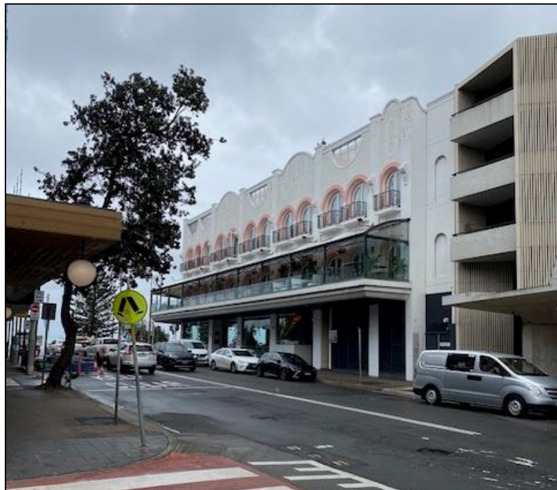
Figure 2: Site viewed from Hall Street
