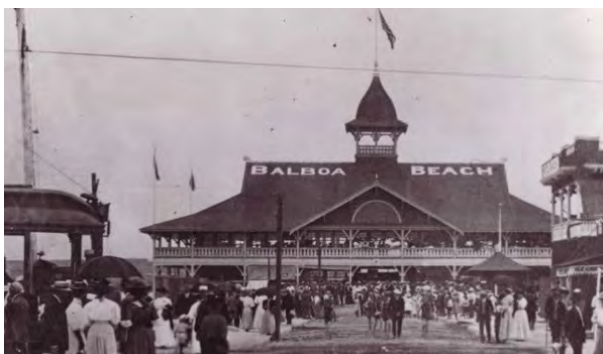
Figure 5.64: Balboa Beach Pavilion, early twentieth century. Source: www.balboapavilion.com
