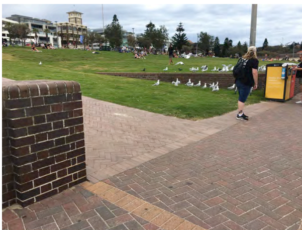
Figure 4.43: The location of the former tunnel entry is where the grass is adjacent the path. All the brickwork is modern. Source: JRA 2020
