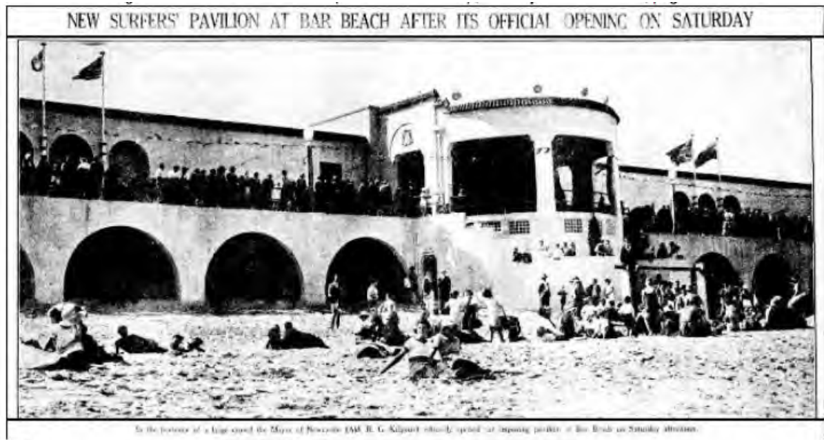
Figure 5.32: Bar Beach Surf Pavilion when completed in October 1933. Source: NHM, 9 October 1933
