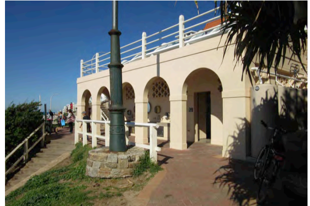
Figure 4.89: Bondi Park South Amenities. This is outside the SHR BBCL boundary. 2016. Source: JRA
