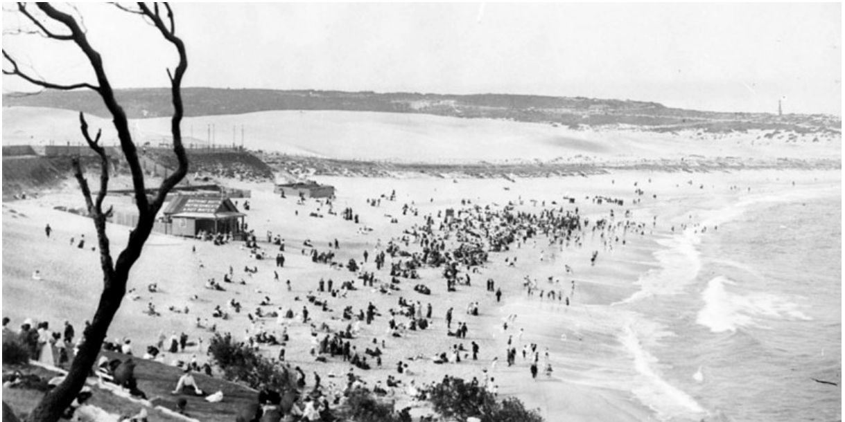
Figure 2.31: c1900 View of Bondi Beach showing the dune system, with grassed terraces and seating in the reserve in the foreground. Note also the tree, that appears dead, curved in the direction of the prevailing wind. On the beach note the refreshment kiosk with writing on the roof (advertising), part of the roof of the surf club (between the tree and the kiosk) and the changing sheds in the mid distance at the base of the tram loop. The dune stabilisation may have commenced with the indistinct line of vegetation behind the beach. Source: ML Hall 35104r
