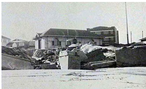
Figure 4.97: Storm damage to the sea wall in front of the Sewage Pumping Station, Feb 1929. Source: WIL 000127
