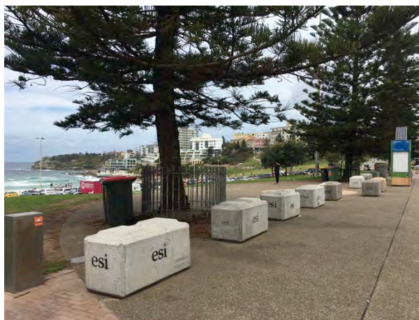
Figure 4.46: Hazard vehicle mitigation barriers installed in 2019 and 2020. Source: JRA
