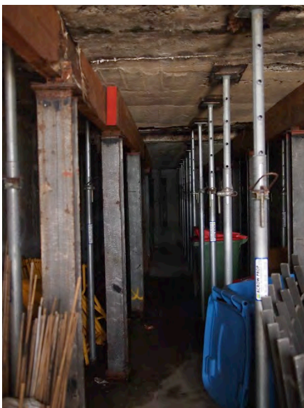
Figure 4.57: Props in Tunnel 1. Source: JRA
