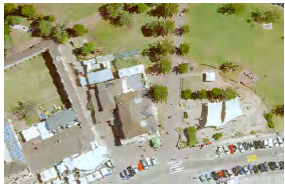
Figure 4.62: 2018 Aerial view of the works depot. Source: Aerial courtesy of Waverley Council
