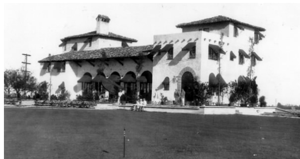
Figure 5.69: American example of a club house, North Palm Beach. Source: http://featured.blog.palmbeachpost.com
