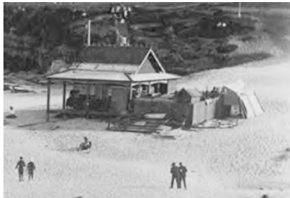
Figure 2.39: c1905 Refreshment kiosk
