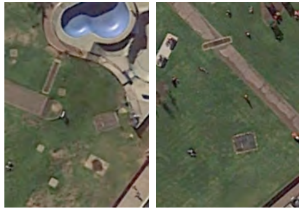
Figure 2.129: 2016 aerial photos showing the stormwater drainage installations. Source: Google Maps
