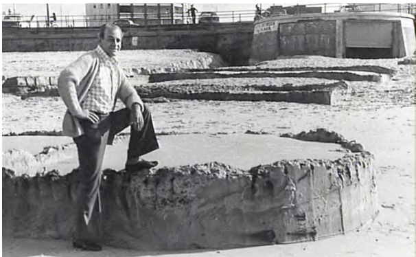
Figure 4.31: Groyne footings exposed after storms in 1974. Source: WIL 000385
