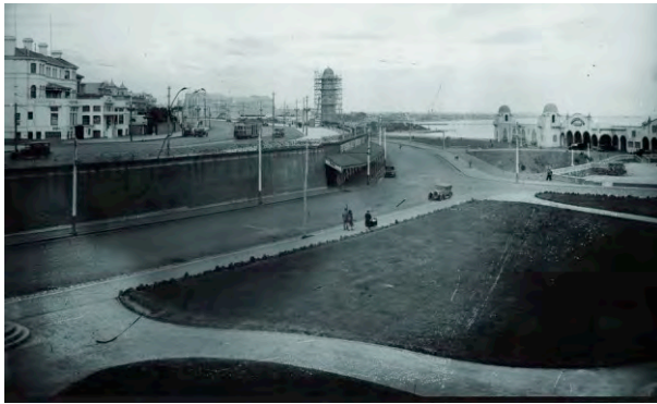
Figure 5.39: St. Kilda beachfront showing the shop fronts that were inset into the large retaining wall behind the beach park, so as to utilise the filled zone constructed to support the main arterial road. Source: St Kilda News
