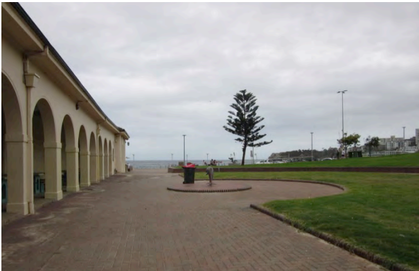
Figure 4.131: Path south of pavilion looking towards beach. Modern paving with raised level. Source: JRA 2020
