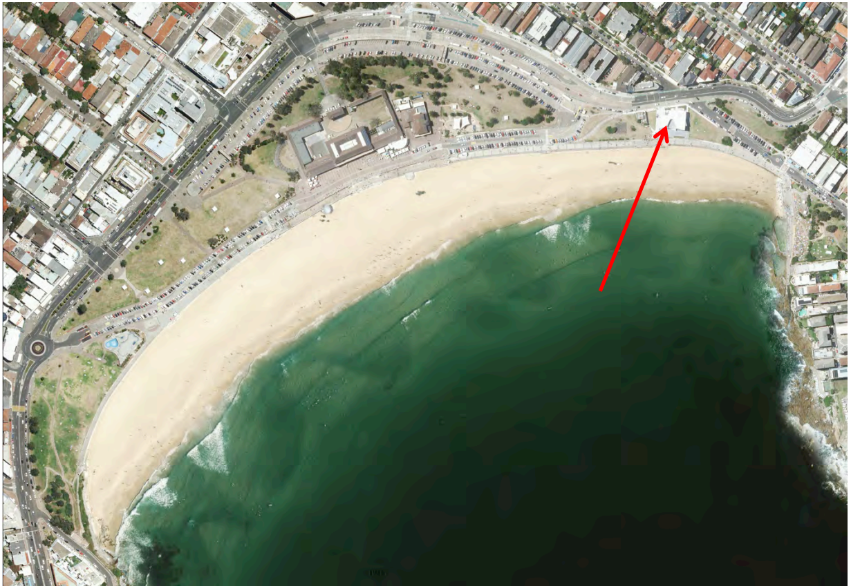
Figure 4.75: 2014 aerial photo. New North Bondi surf club (arrowed red). Source: Waverley Council
