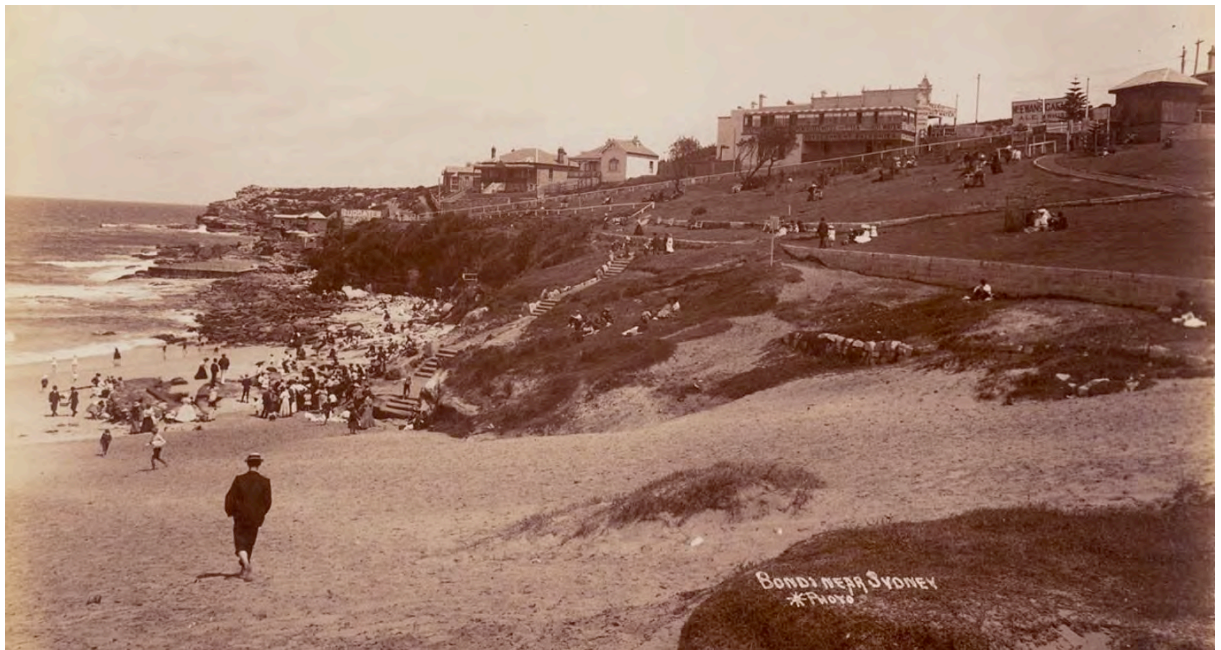
Figure 2.27: c1900 - 1910 View of Bondi Beach showing the improvements made to the reserve at the southern end of the Beach. Stone retaining walls form grassed terraces accessed by paths and stairs. Some remnant indigenous plants survive at the top centre of the photo and a Norfolk Island pine is visible adjacent the tram shelter (top right). This is one of the earliest Norfolk Island line plantings at Bondi. The baths can be seen at left in the middle distance. Source: Star Photographs, ML digital order number a116186h, PXE 711/186
