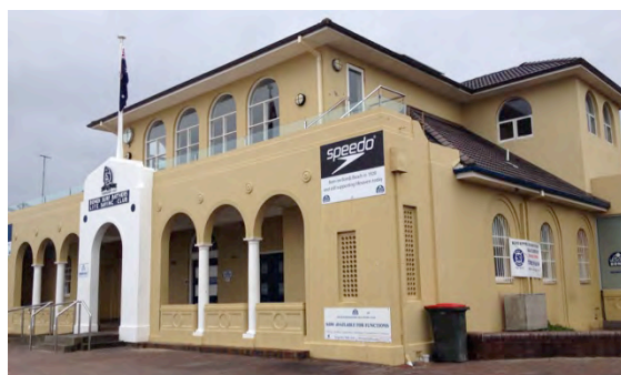
Figure 4.60: The BSBLSC, showing the first floor addition and the east entry addition on the right, 2015. Source: JRA
