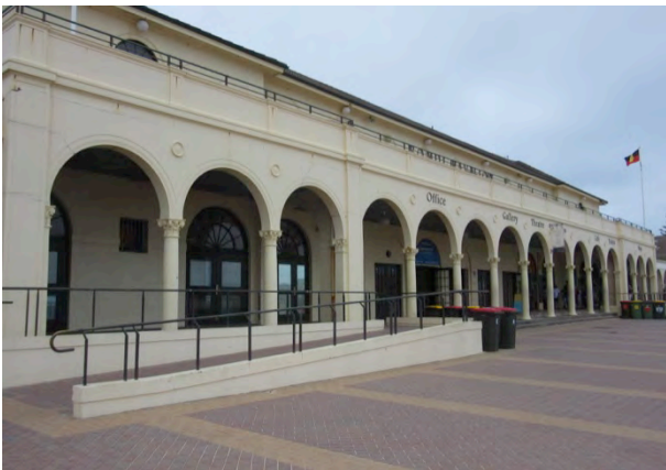
Figure 4.129: Close view of the pavilion arcade. The modern paving is raised. Disabled ramp on left. Source: JRA 2020
