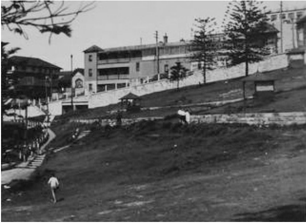
Figure 4.92: The Balconies, Bondi Beach. The retaining wall to Notts Ave looks newly built. Postcard sent c1941. Source: NMA Josef Lebovic 1986.0117.7182
