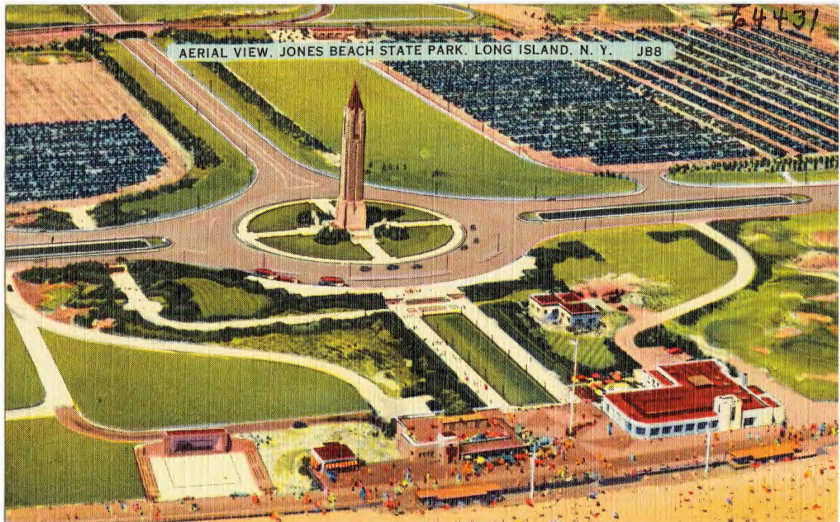
Figure 5.24: Jones Beach State Park, Long Island, New York completed in 1929 showing the underpasses from the Parking Fields. Source: www.digitalcommonwealth.org
