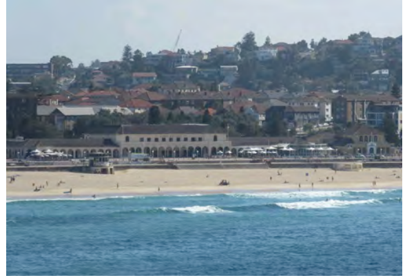
Figure 4.56: Distant view of Surf Pavilion 2015. Source: JRA
