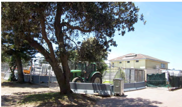
Figure 4.61: View of the works depot at the rear of the BSBLSC in 2016. The fencing and equipment in the foreground have since been removed. Source: TZG
