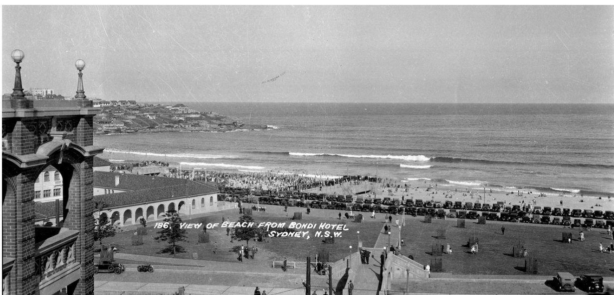
Figure 2.71: c1930s. One of Samuel Wood's views of the Bondi Beach Improvement Scheme taken from the Bondi Hotel showing the motor park and pedestrian bridges and the arcade to the southern side of the pavilion. Newly planted trees are visible protected by tree guards and three more mature pine trees on the left. Source: ML digital order a1470145
