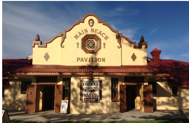
Figure 5.72: Main Beach Pavilion in 2014. Source: JRA
