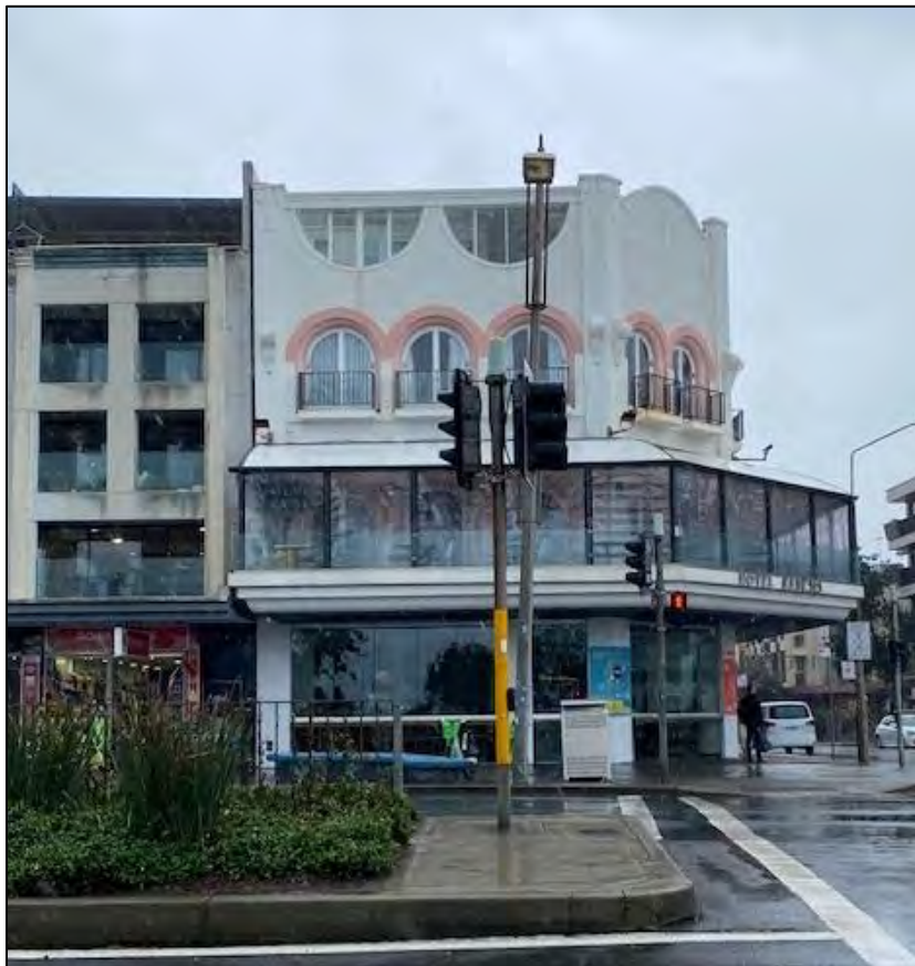
Figure 2: Site viewed from Campbell Parade looking west.
