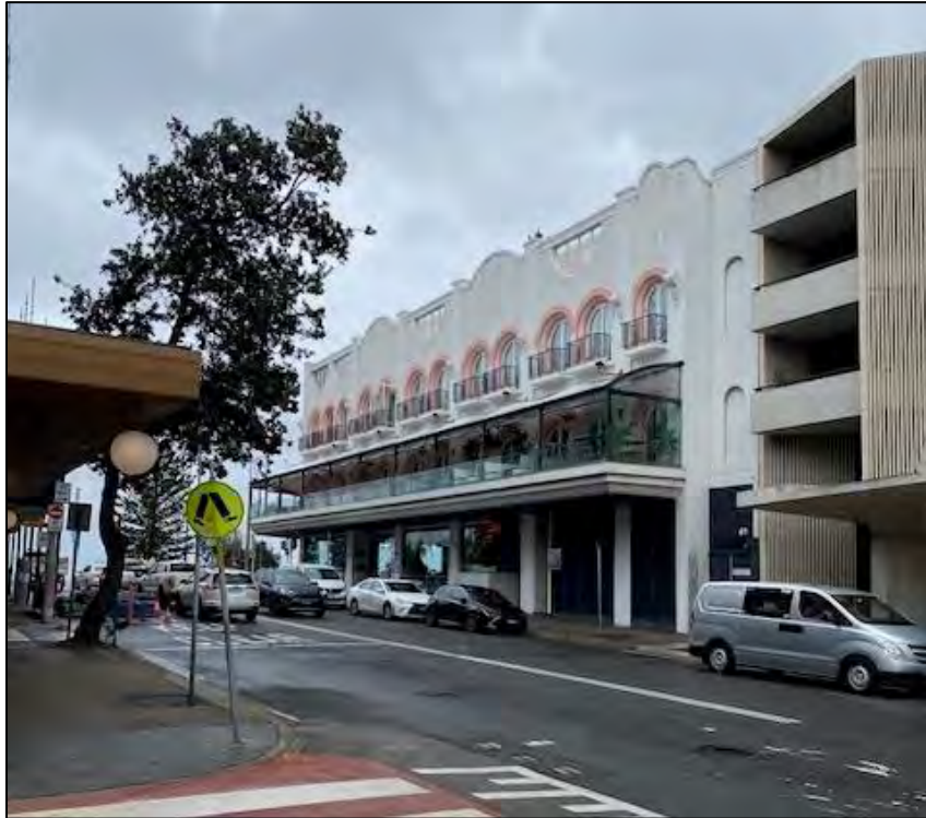
Figure 3: Site viewed from Hall Street looking east.
