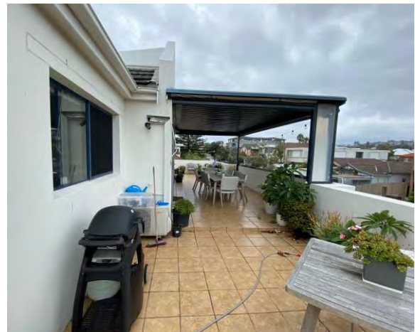
Figure 6: Westerly view of the existing vergola to Unit 8.
