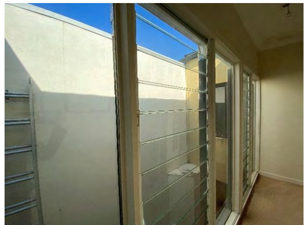
Figure 6: Existing void at the first floor.
