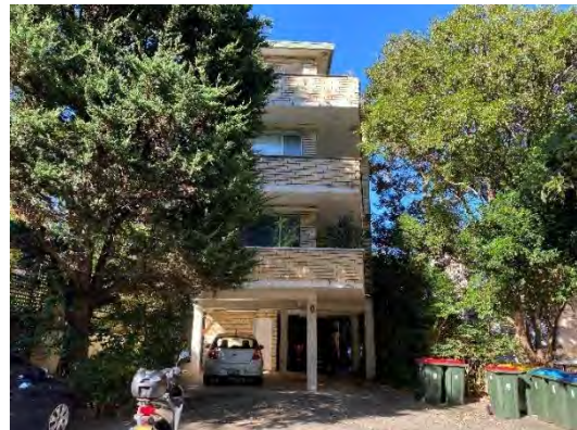
Figure 2: View of the existing building from Arnold Street.
