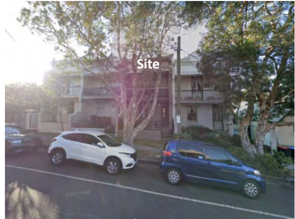
Figure 2: View of the site context.
