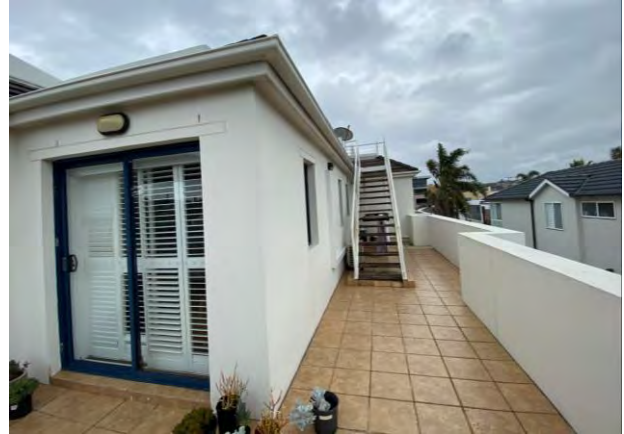
Figure 2: Western staircase from Unit 8 to the roof terrace.
