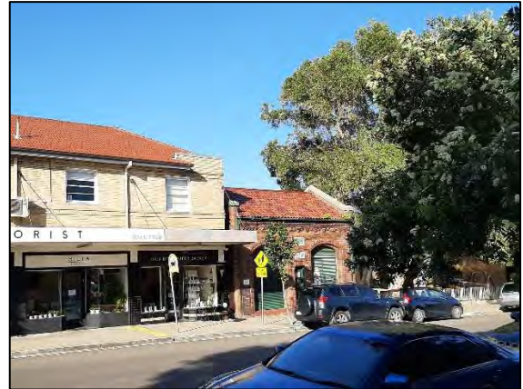
Figure 6: Heritage listed substation adjoining the west of the site
