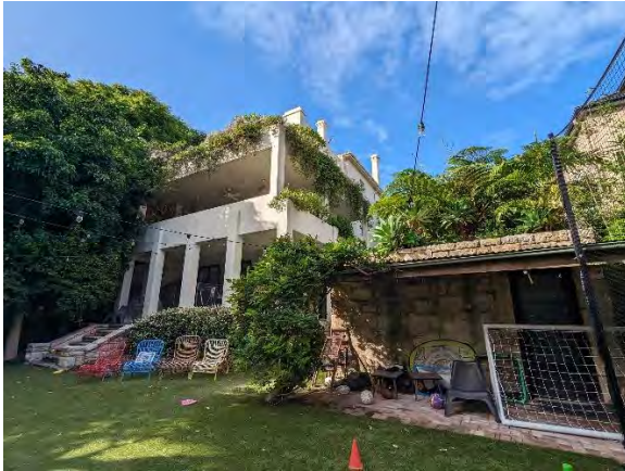
Figure 5: Rear of subject dwelling house viewed from rear yard looking south-east
