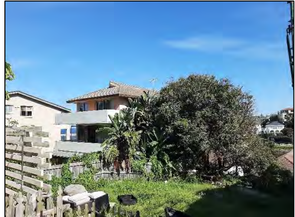
Figure 2: Rear elevation of the building as viewed from Silva Street.
