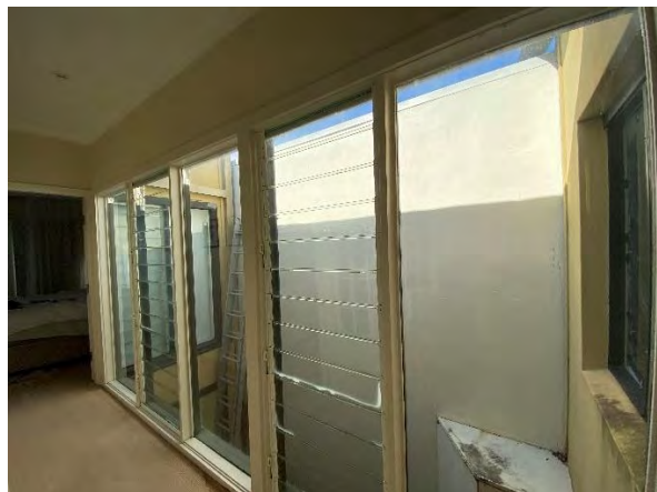
Figure 5: Existing void at the first floor.
