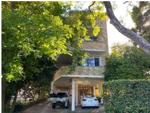
Figure 1: View of the existing building from Queens Park Road.
