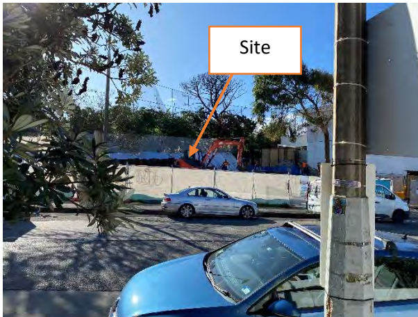
Figure 1: Streetscape view of the subject site
