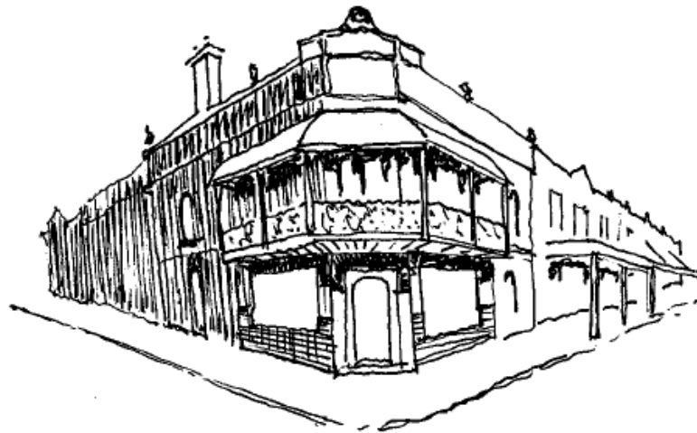
Figure 15 Original verandahs should be retained
