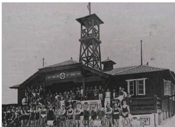
Figure 2.53: North Bondi SLSC timber building, c1920. Source: Digital Masters, NBSLSC
