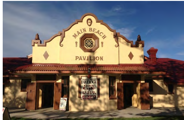
Figure 5.72: Main Beach Pavilion in 2014. Source: JRA
