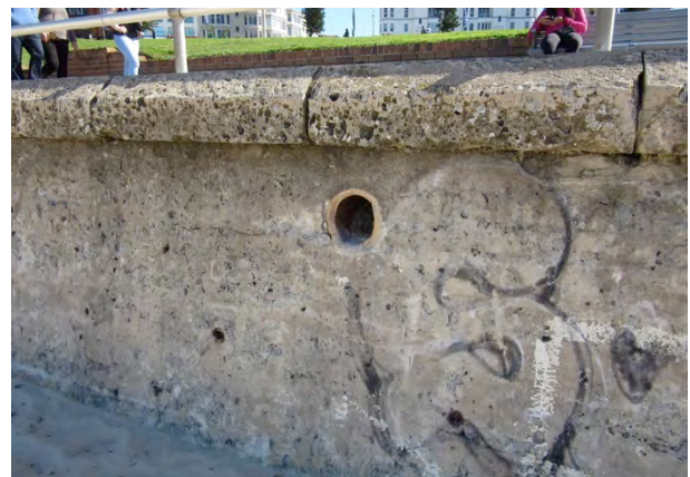
Figure 4.35: Sea wall showing one of the earthenware drains probably now obsolete, 2016. Source: JRA
