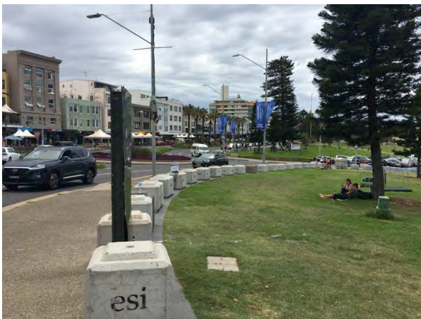
Figure 4.90: Concrete hazard mitigation blocks near the roundabout. Source: JRA 2020
