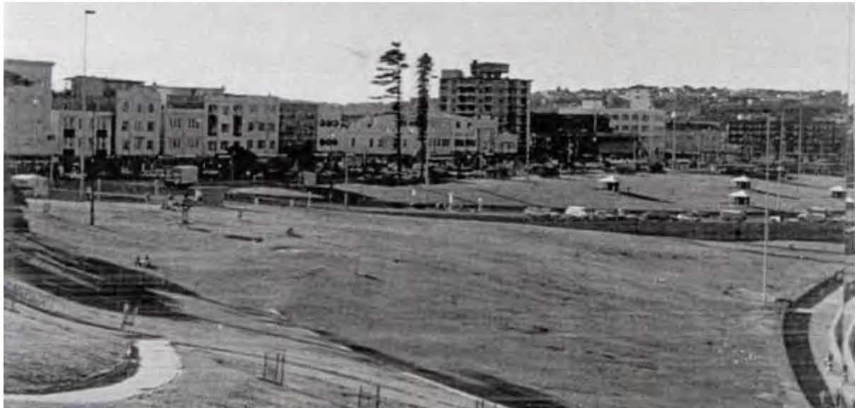
Figure 2.120: In 1986 upgrades had commenced with picnic shelters built for shade and ground levels raised with a retaining wall on the upper side of Queen Elizabeth Drive and above the promenade at the right of the photo. There are no trees except two surviving earlier Norfolk Island pines at the centre and a group out of the photo to the left (shadows). The path across the end of the park is visible just to the left of the two pines. Source: WIL 102122
