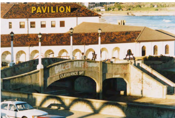
Figure 5.37: Bondi Park footbridge and lamps. Source: WIL 000307
