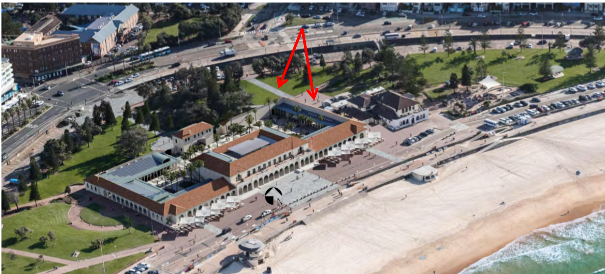
Figure 7.9: Extract from 2019 DA architectural drawings by TZG. Most of the changes are within the pavilion footprint. The new access road and paved turning area can be seen behind the surf club (arrowed). Source: Waverley Council
