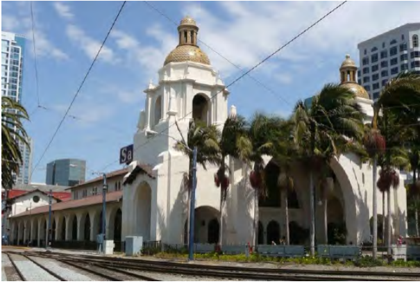
Figure 5.66: San Diego Railway Station (Santa Fe depot). Source: http://harvey-house.info/california_2
