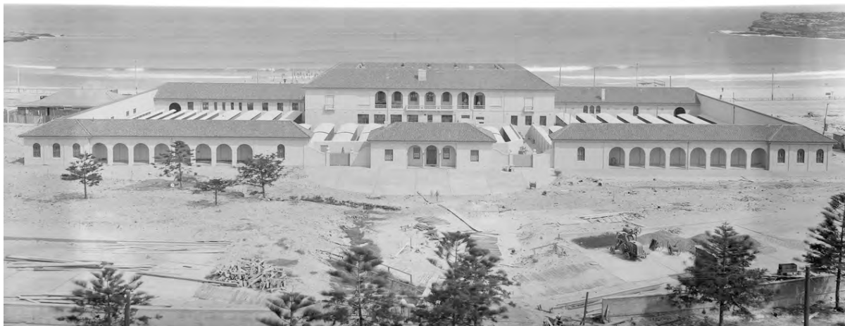
Figure 4.53: The Surf Pavilion prior to completion of landscaping works, 1929. Note the Norfolk Island pines from earlier plantings. Source: SL NSW a6879025, Arthur Ernest Foster
