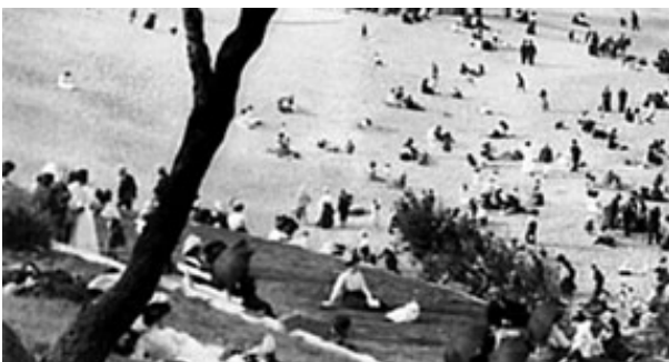
Figure 4.86: Extract from a historic view showing the grassed terraces and park benches. Source: ML hall 35104r
