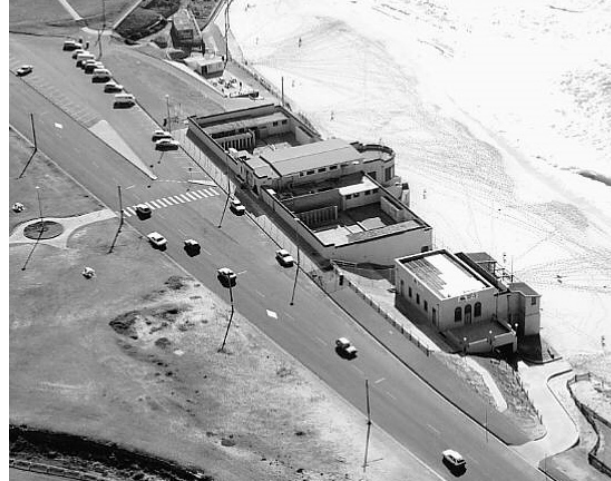
Figure 5.63: Bar Beach Pavilion, Newcastle in 1939, since substantially demolished. The road works were undertaken as an Unemployment Relief Scheme project.
