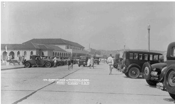
Figure 4.77: This early c1930 photo shows the concrete panels extending to the kerb. Source: ML a1470110h
