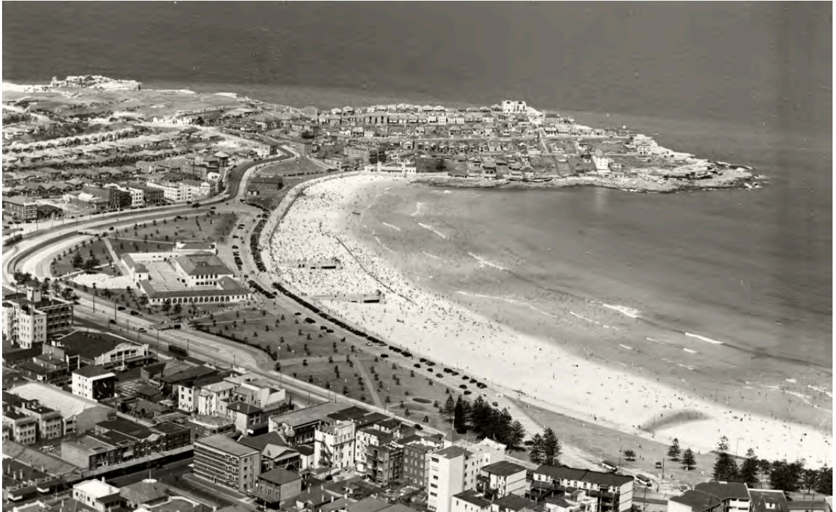
Figure 2.67: Mid 1930s view of the improvement scheme showing the surf pavilion in the centre, the marine drive, motor park, promenade and the groynes. Also shown are the low level sewerage pumping station, the two new surf clubs and the grassed Scarborough Bank. The layout of the plantings can also be seen, including the mature Norfolk Island pines at the southern end of the beach planted before the improvement scheme. A diagonal path has been added south of the pavilion. Source: Adastra Aerial Survey 1937, RAHS via Flickr
