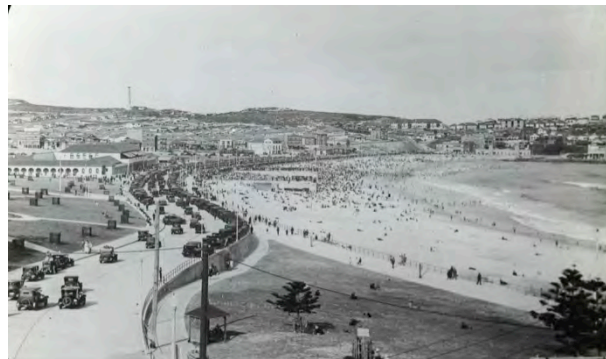
Figure 4.78: Photo c1930 showing the newly completed roadway and retaining wall. Source: SLVIC H92.350/35
