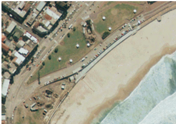
Figure 2.128: 1991 aerial image showing excavations for stormwater drainage improvements. Source: Aerial courtesy of Waverley Council
