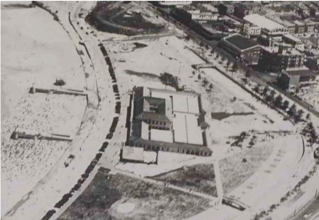
Figure 2.65: 1928 view under construction. The marine drive is completed except where obstructed by the tram loop and there is still road access across the park just north of it. The motor park and bridges are built and some paths. Some of the older Norfolk Island pine plantings remain on Campbell Parade but plantings have not been made in the park. Source: Ari Anderson
