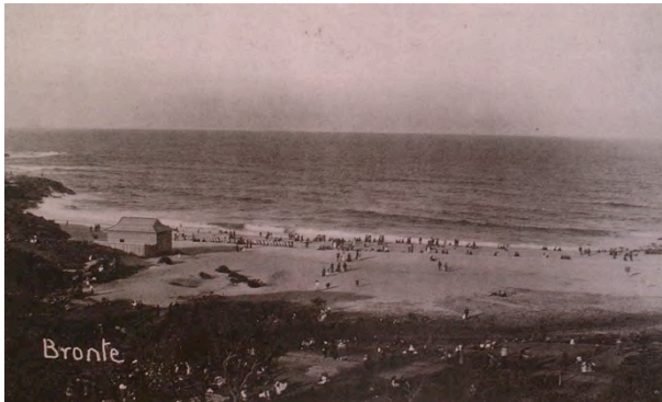
Figure 5.16: View over Bronte Beach c1910, showing the recently completed first SLSC. Building at left. Note that the park has not been filled in and levelled by this time. Image courtesy of Mr Robert Mills. Source: AA
