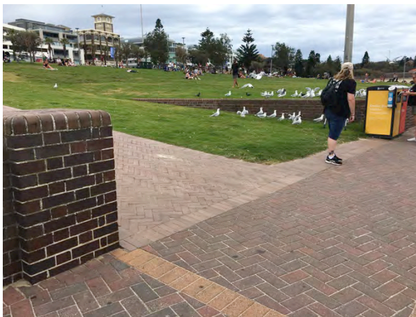
Figure 4.43: The location of the former tunnel entry is where the grass is adjacent the path. All the brickwork is modern. Source: JRA 2020
