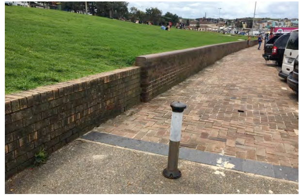
Figure 4.42: Junction of blond brick wall and later dark brick wall along QED and a section of original herringbone pattern paving in light brown common bricks. Source: JRA 2020
