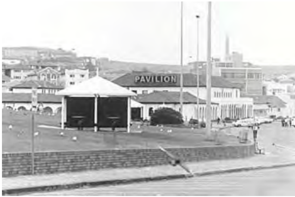
Figure 4.41: 1981 view showing the first generation brick retaining wall along QED and the then new picnic shelter. Source: WIL 000302
