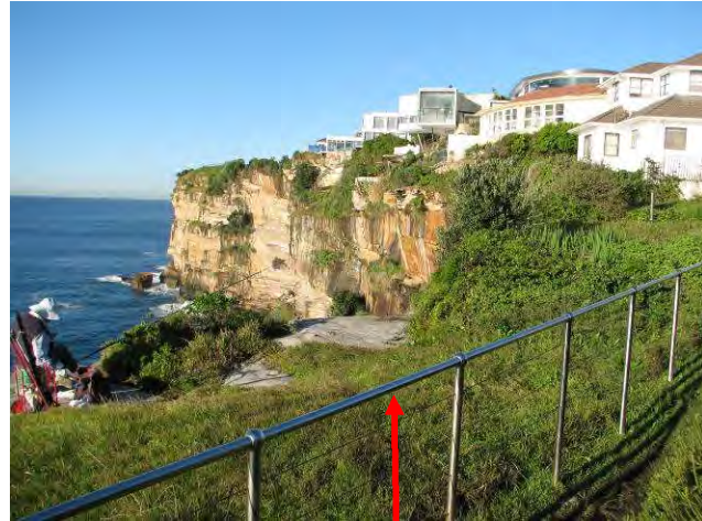
Eastern end of Lancaster Road
