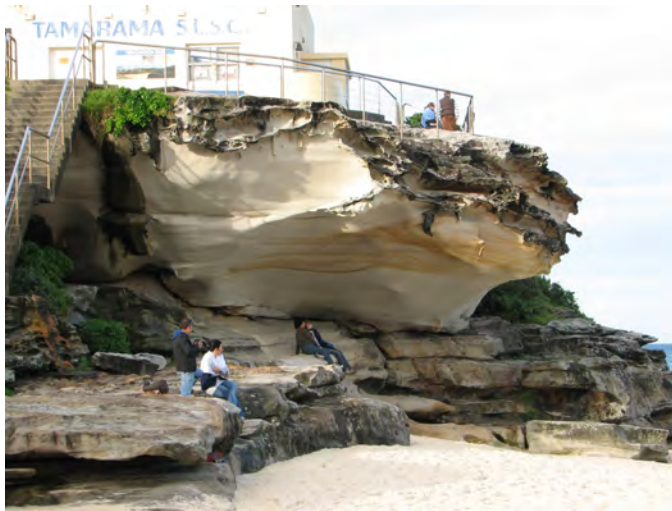
Figure 5.3 Cliff top overhang and undercut features
