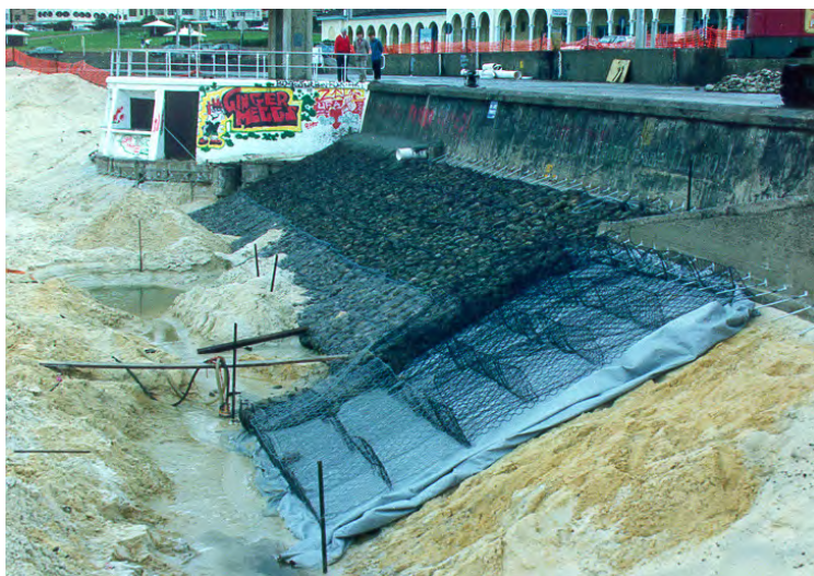
Figure 2.11 Construction of Bondi Seawall, Reno-mattress toe protection works 1987 (Source: Lex Nielsen)
