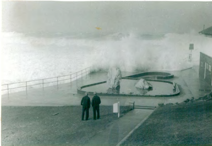
Figure 3.12 Overtopping at Bronte, 1974 (source: Waverley Council)
