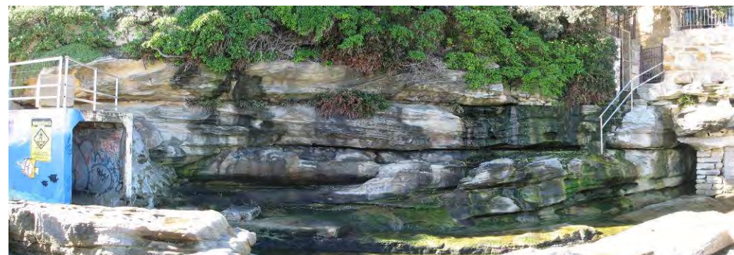
Stormwater box culvert
