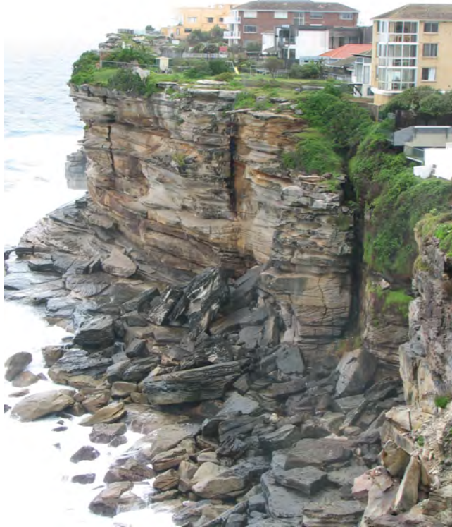
Figure 5.1 Cliff face failure onto wave cut platform
