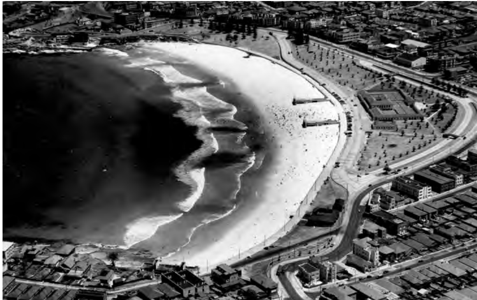
Figure 2.7 Aerial photograph showing piers, 1940 (source: Waverley Council)
