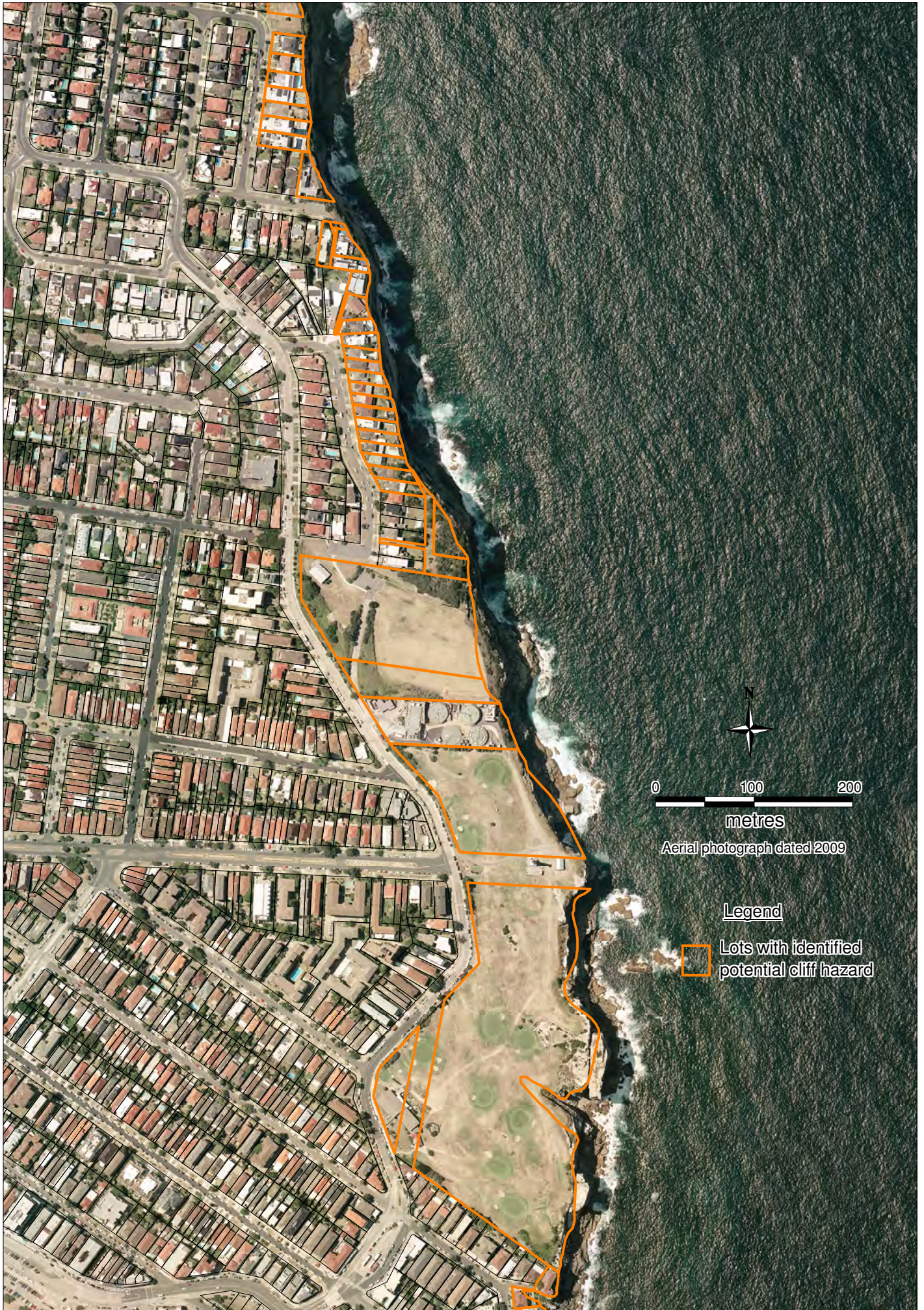
LOTS WITH IDENTIFIED POTENTIAL CLIFF HAZARD (3 OF 6)
