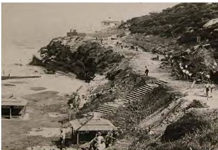
Figure 2.20 Tamarama, 1931, construction of Marine Drive. The seawall and picnic huts can be seen (Source: Waverley library)
