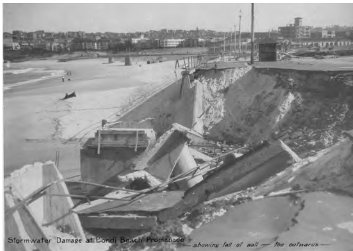
Figure 3.15 Bondi Northern Seawall Failure, 1929 (Source: Waverley Council)
