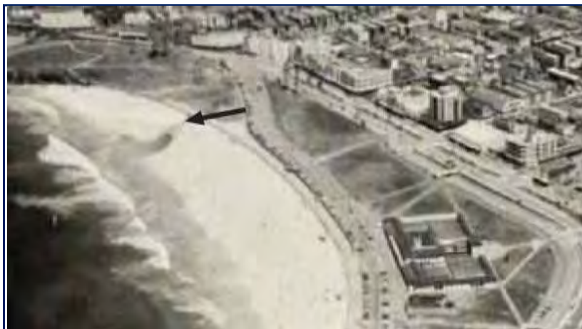
Figure 3.2: Stormwater drainage crossing the beach in 1972. This general location, at the southern end of the beach, may be within the vicinity of the delta seen in 1899 (Mayne Wilson & Associates 2012: Figure 57)
