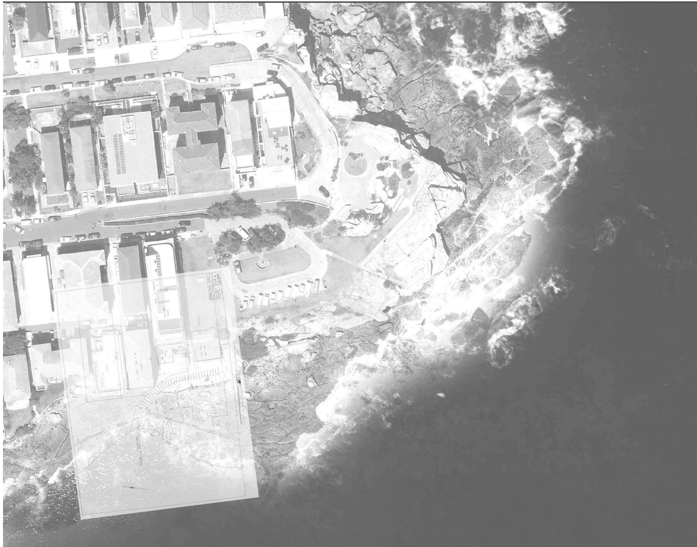
Waverley Municipal Council Boat Ramp to Ben Buckler Fishing Club at Low Tide WLS Index No. 855
