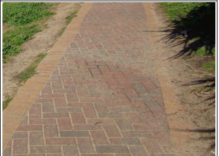
Modern path between retaining walls from the near QED to the Toilet Block – herringbone brick with soldier course to the edges. Source: JRA
