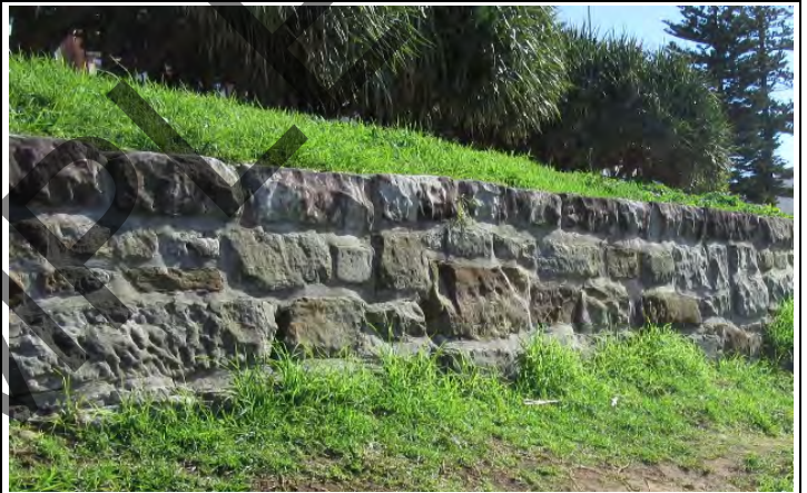
Sandstone Retaining Wall – roughly coursed rock face sandstone. Source: JRA
