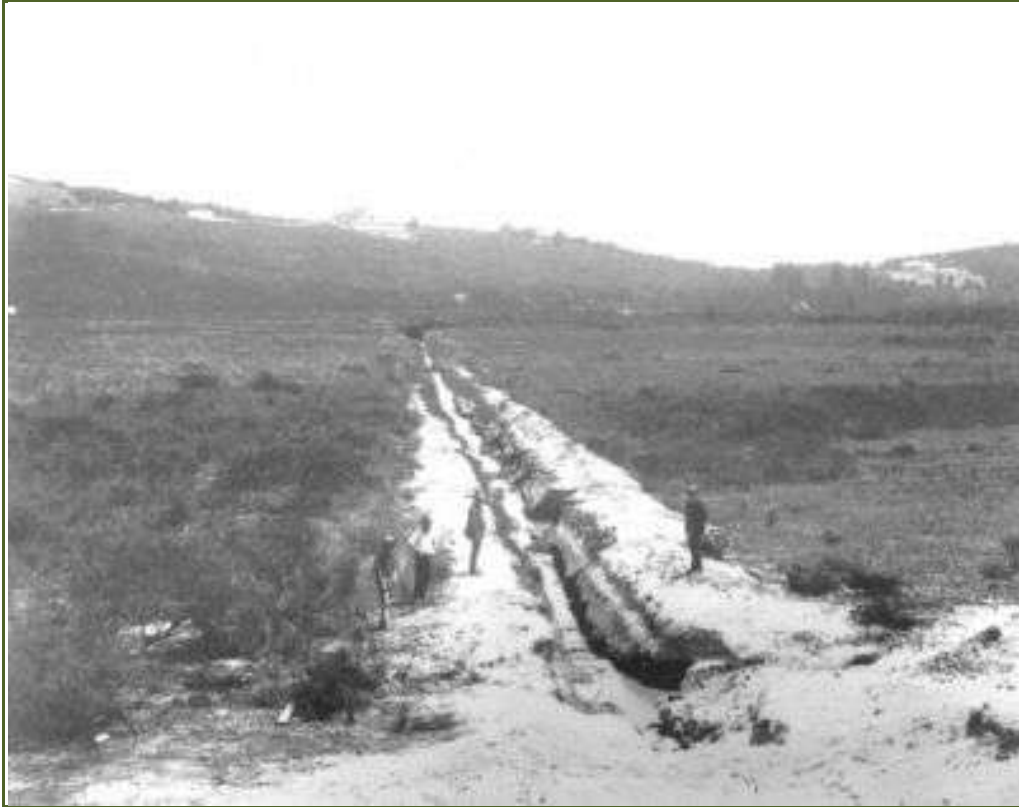
Figure 2.16: This section of the Bondi Ocean Outfall Sewer was oviform and brick lined (Water NSW)
