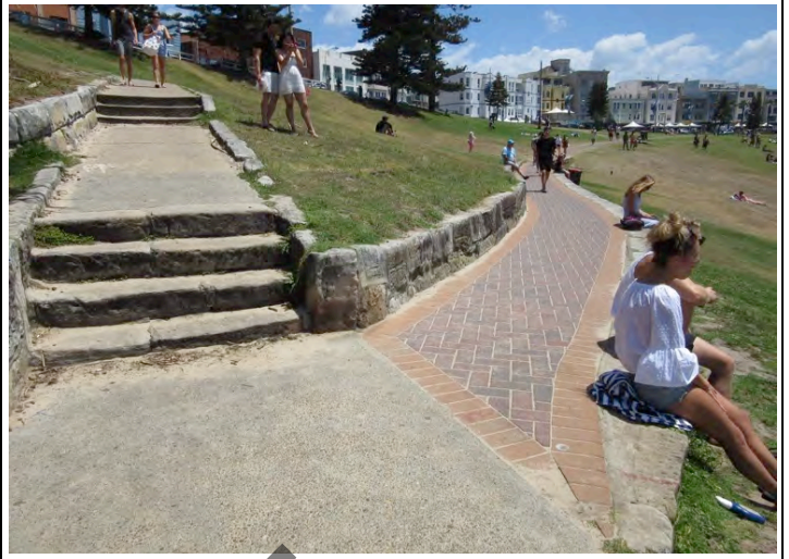
1894 sandstone steps and path with stone edging. The right path and the retaining wall above it is modern but the wall below is 1894. Source: JRA
