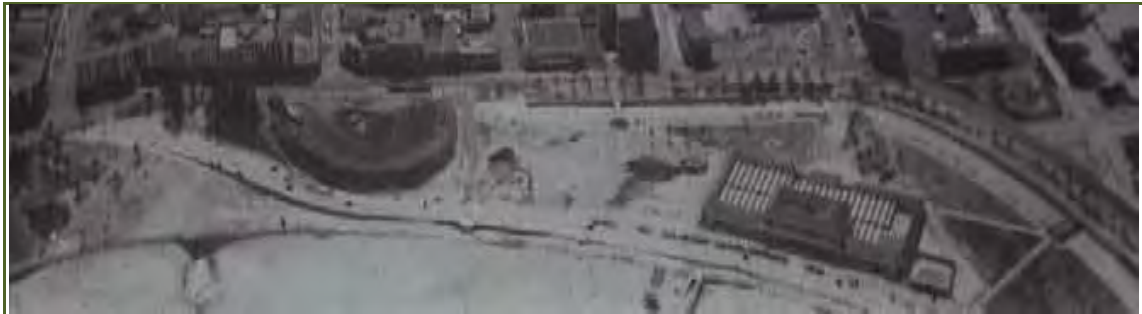
Figure 4.7: Bondi Beach in late 1928 showing the Pavilion under construction (TKDA 2015: Figure 19)
