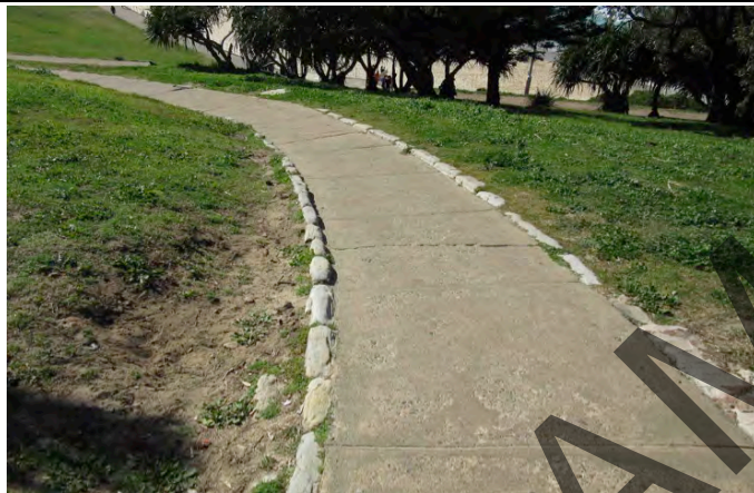
Zig Zag Path – Concrete panels with sandstone edging. Source: JRA
