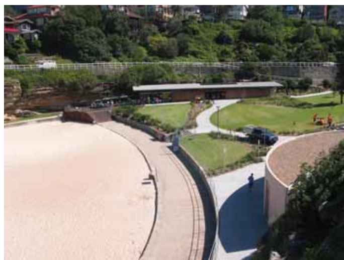
Amenities building and kiosk, Tamarama Park
