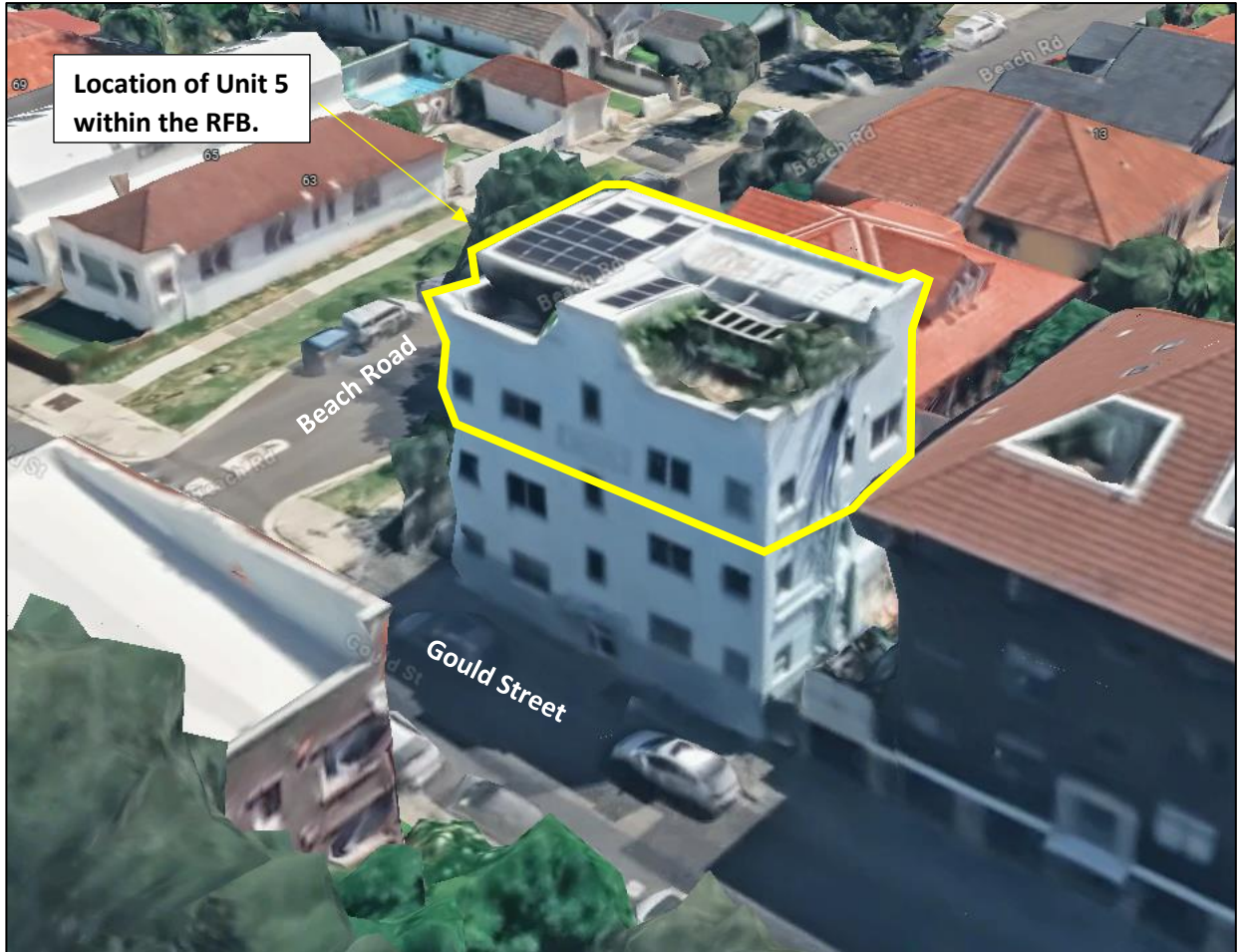
Figure 1. Subject unit and surrounding urban context, looking west. (Source: Google Maps, 2024)
