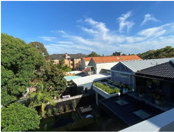
Figure 33. Properties neighbouring to the northwest. Image obtained from the DA-366/2022 Assessment Report.
