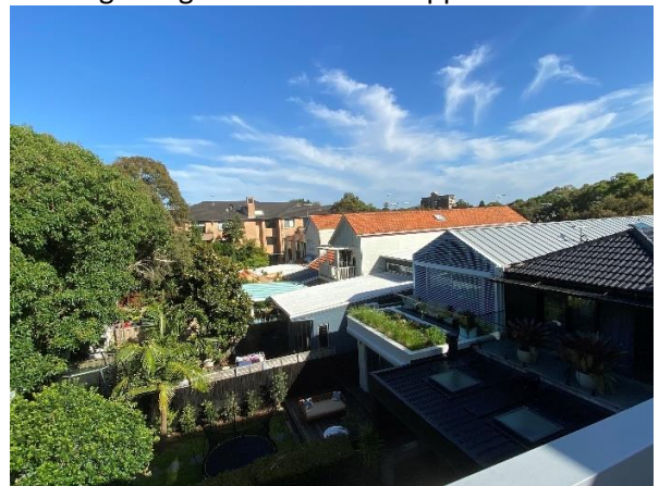
Figure 6: Rear setbacks of the properties neighbouring to the northwest. Image obtained from the DA-366/2022 Assessment Report.
