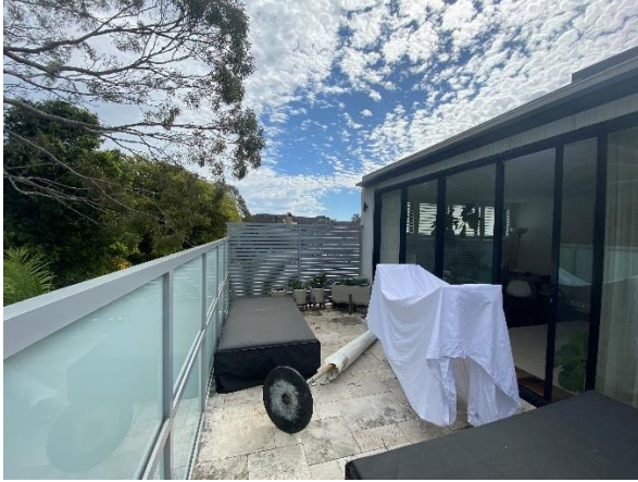
Figure 31. Level 2 balcony facing northwest.
