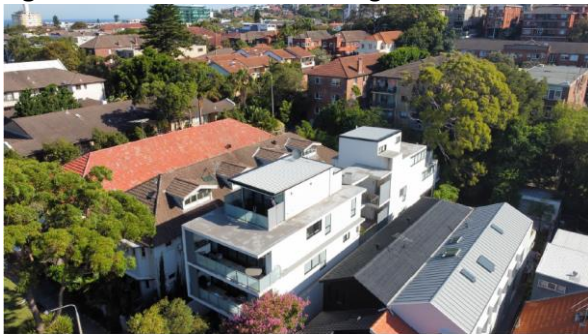
Figure 3: South facing aerial view of the building. Image obtained from applicant's SEE.
