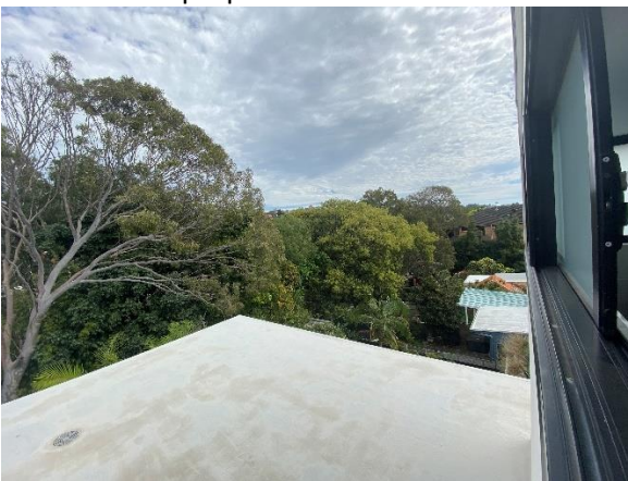
Figure 9: View from the attic level bathroom window of the subject unit looking west where the works are proposed.
