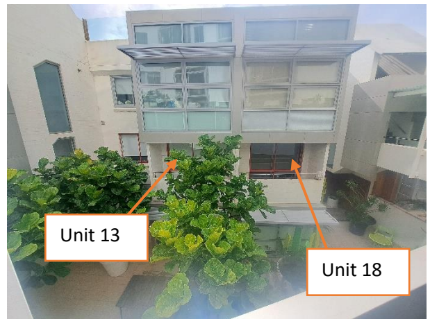
Figure 4: Rear view terraces of Unit 13 and Unit 18
