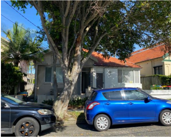
Figure 1: Westerly view of the front façade of the subject sites from Nancy Street.
