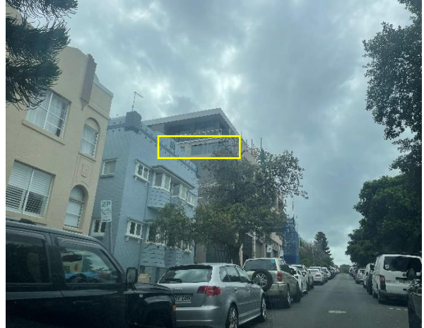
Figure 2: Subject site, viewed from Ramsgate Avenue looking north-west. Proposed location of works is outlined in yellow.
