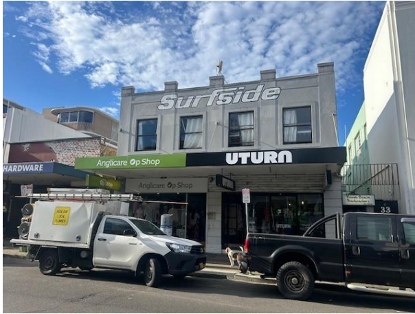
Figure 1: Site frontage, No. 35-37 Hall Street, facing north.
