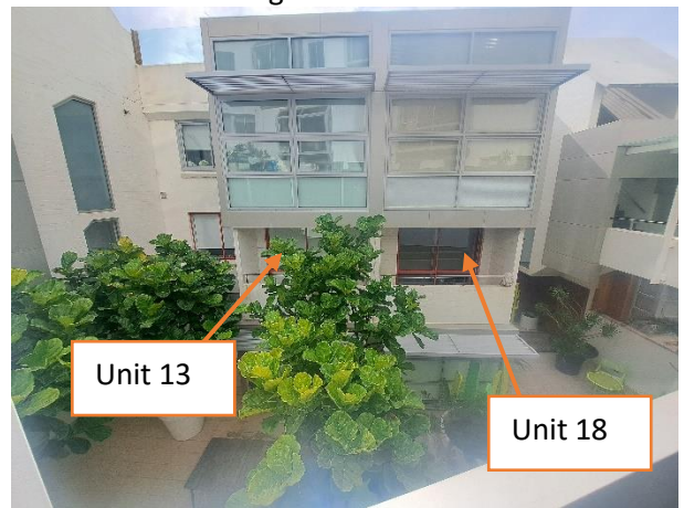
Figure 4: Rear view terraces of Unit 13 and Unit 18.
