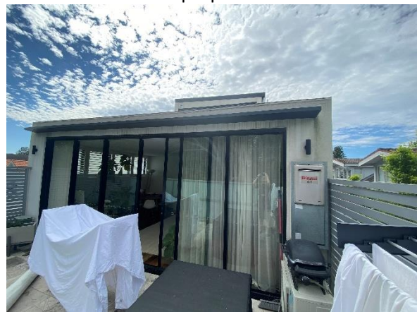
Figure 10: Rear of level 2 facing north.
