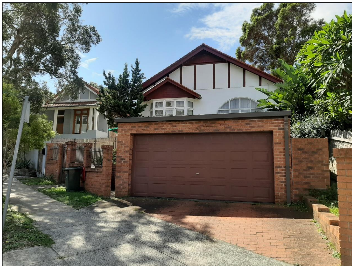
Figure 1: Site viewed from Lamrock Avenue.
