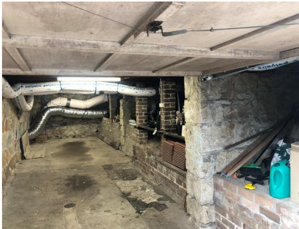
Figure 7: Existing garage, looking south
