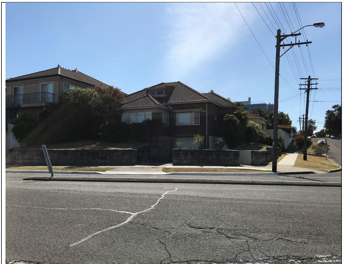
Figure 1: Site viewed from the corner of Military Road and Dover Road looking east
