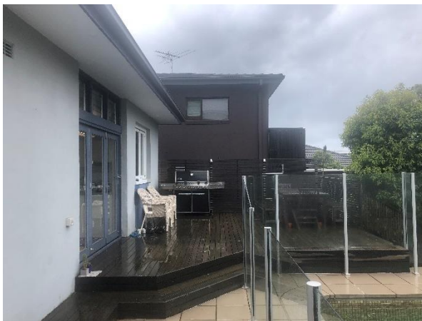
Figure 3: Existing rear deck and adjoining dwelling (28 Yanko Avenue), looking east
