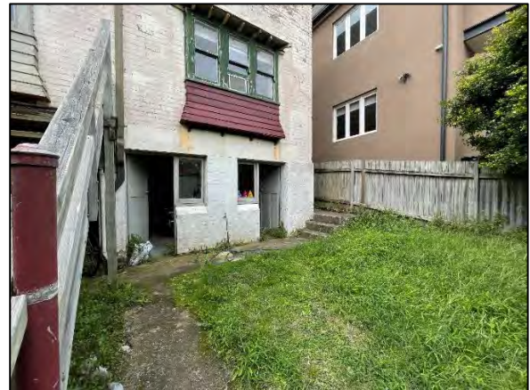
Figure 4: Rear of existing building including subfloor space to be converted to a new unit, looking northeast.
