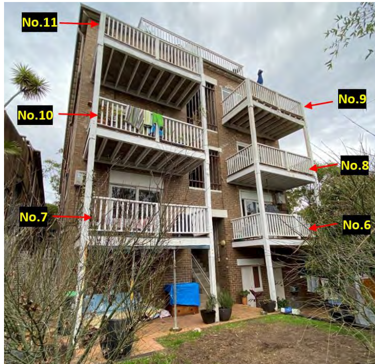
Figure 1: Site viewed from rear side of the building (north-eastern side)
