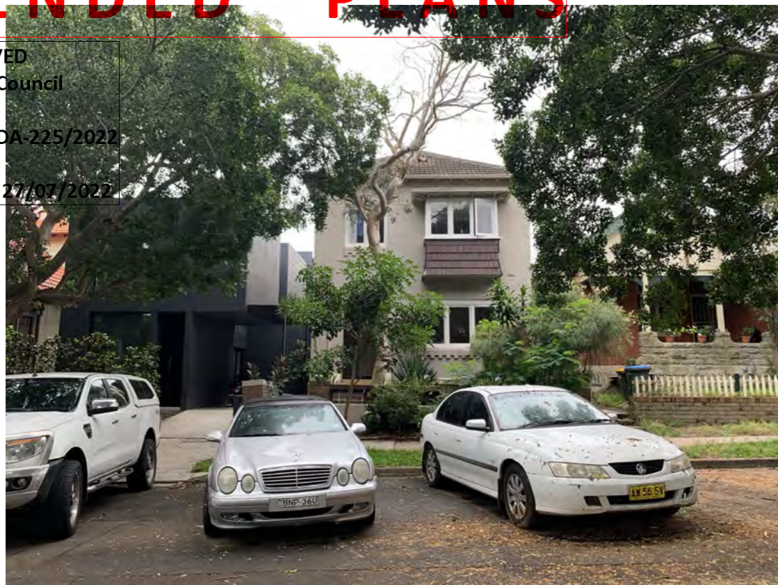
1 Street View Front - Existing
