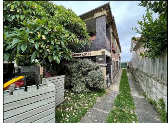
Figure 2: Western side boundary leading to the detached garage at the rear.
