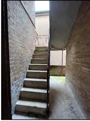
Figure 7: Existing fire stairs in eastern side boundary to be demolished.
