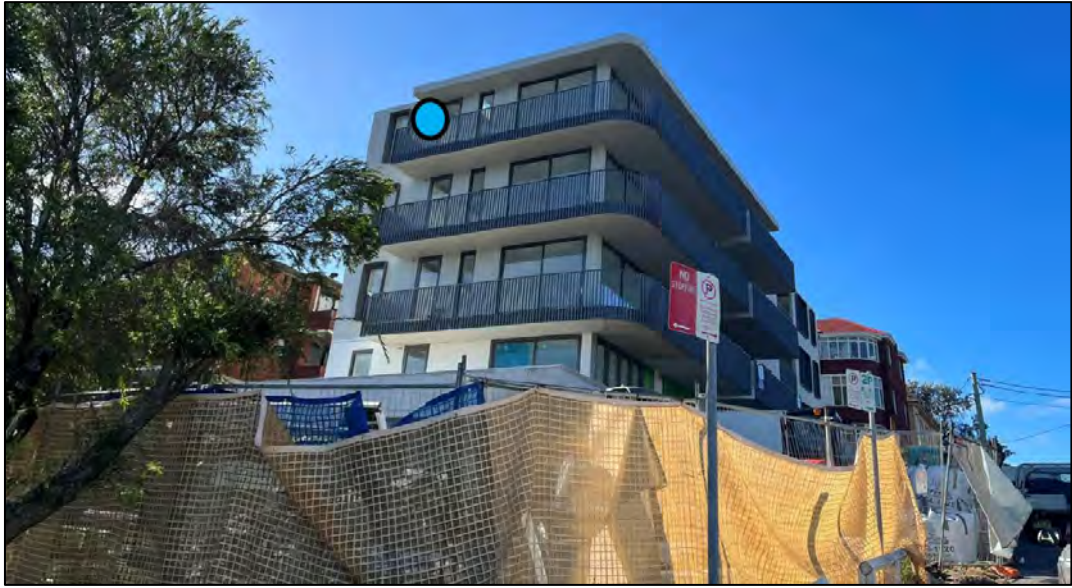
Figure 16: Southern elevation of 14 Fletcher Street indicating location of analysis (level 4). Source: Navon Planning.
